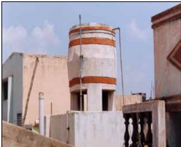
Figure 2. Inaccessible overhead storage tank in Chennai (photo courtesy of Dr Rajander Sharma)
