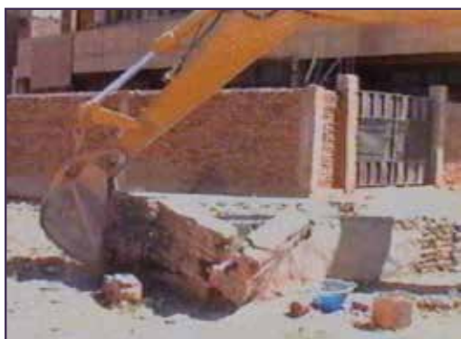
Figure 2. Removal of water basins (photo courtesy of KMFJ)
