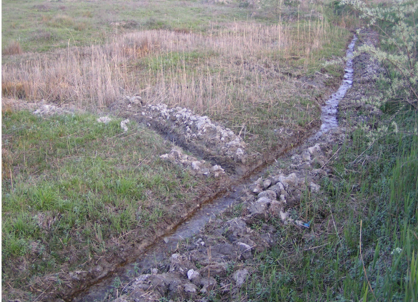
Fig. 23. Small hydraulic engineering in Kadamzhai district, Batken province, 2004: the channels helped to divert water and drain the swamp
