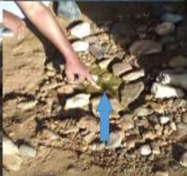
Water seepage from tap running in the ditch
